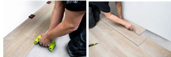
10. Fit the second row as you did for the first: start on the left hand side and slide the groove of the panel under an angle of about 25° over the tongue of the previous row, clicking the groove into the tongue by laying down the panel while pushing it firmly against the first row. Along the long edge, it is advisable to use a recoil or rubber hammer and tapping block, or cut piece of panel profile to tap the panels tightly together and to ensure the click mechanism is firmly locked.
