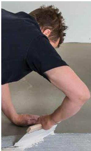
For the installation of Xtrafloor® Flex Pro: lay the sheets butted, edge-to-edge, at a 90 angle to the laying direction of the new floorcovering. Xtrafloor® Base and Xtrafloor® Flex-Pro is to be laid PET Film side up and Xtrafloor® Silent is to
