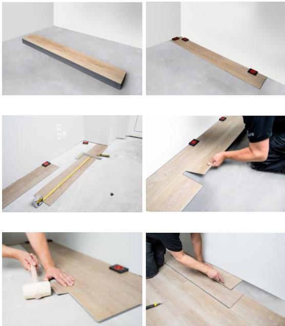
12. To fit the last row of panels you will usually need to narrow them. Do this as follows: lay a panel on top of the previous row with the groove towards the wall, lay another panel upside down up to the edge of the wall and mark the panel underneath. Cut the panel to size and fit the last row.
