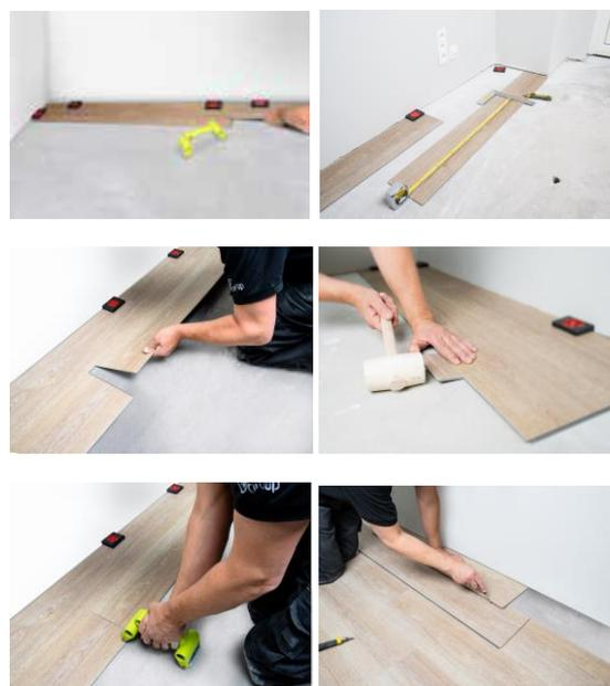
10. Fit the second row as you did for the first: start on the left hand side and slide the groove of the panel under an angle of about 25° over the tongue of the previous row, clicking the groove into the tongue by laying down the panel while pushing it firmly against the first row. Along the long edge, it is advisable to use a recoil or rubber hammer and tapping block, or cut piece of panel profile to tap the panels tightly together and to ensure the click mechanism is firmly locked.
