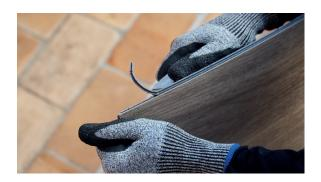
Put the panel with cut-off sides against the walls. Use the spacers to fill out the contour of the wall so that the panels do not move, are straight and are 100% installed and locked together correctly.
