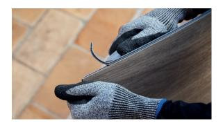
Put the panel with cut-off sides against the walls.
