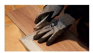
In places where it is too difficult to install the EVF Uniclic® panels with the tapping block (e.g. against the wall), you can tap them together using the pullbar and a hammer.
